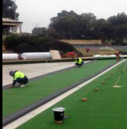
Boddington Bowling Club construction - DryMax Pro
